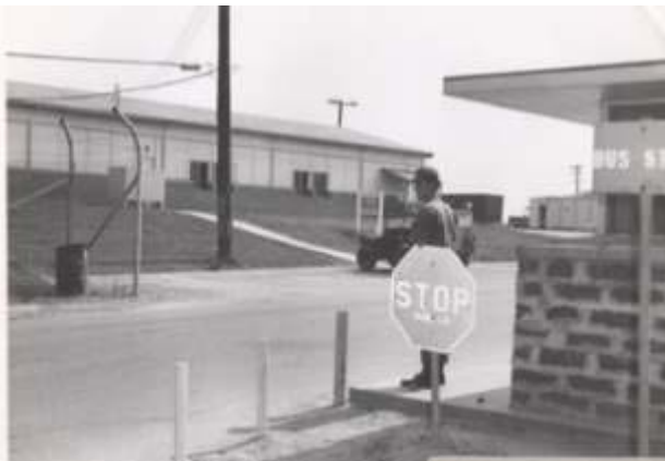
1969 photo of Phu Cat flightline gate with 37 th SPS headquarters in the background (Security Forces Museum)
